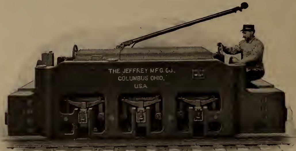
JEFFREY T.M. 150 20-TON ELECTRIC MINE LOCOMOTIVE DRAW BAR PULL 8000 LBS.
